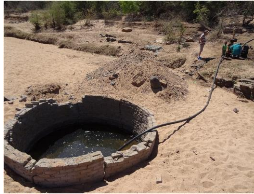
Riverbed well Molototsi sand river in October 2016 during a drought (Walker et al. 2018)
